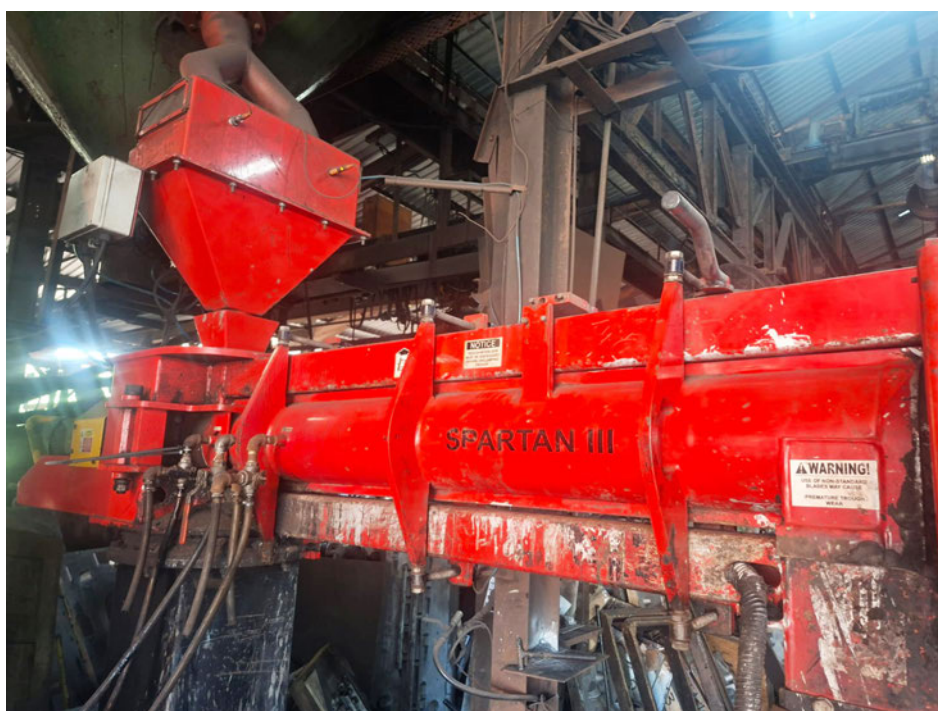
“Just over a year ago we modernised our sand mixing equipment with the installation of an Endeco Omega Sinto continuous mixer. Our chemical supplier supported us in acquiring the 10-ton an hour continuous mixer.”
